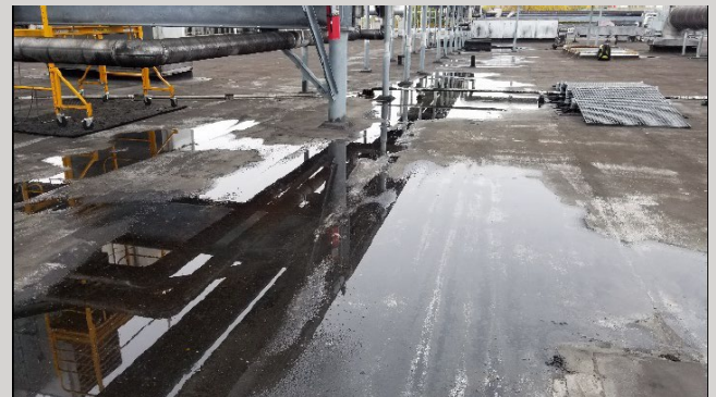
Roof Area B – Partial overview of roof area; ponding water over primary east/west corridor
